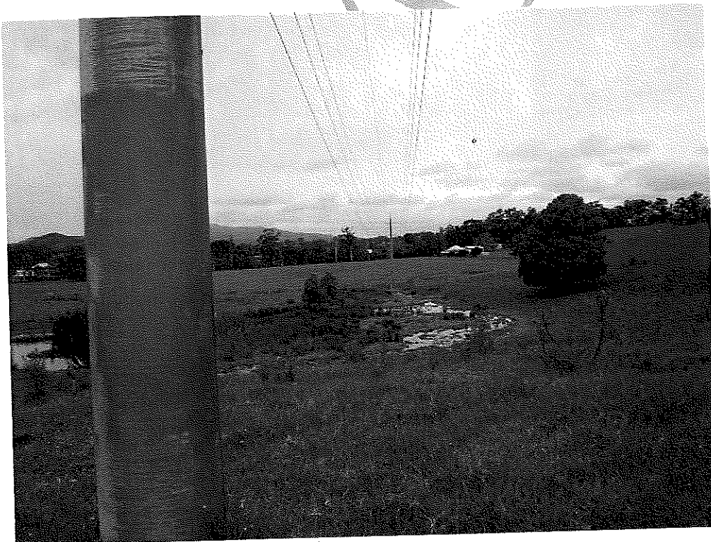
Looking south along line of transmission lines
