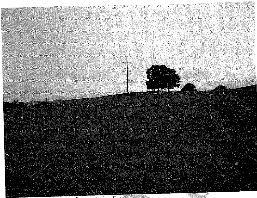
Looking south along line of transmission lines
